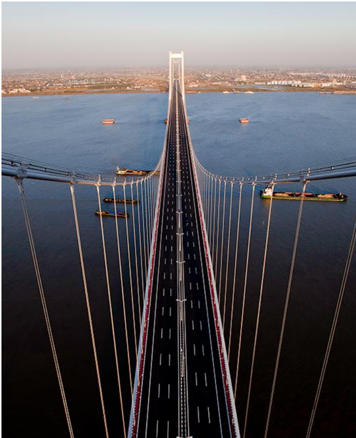
The Taizhou Bridge in Taizhou, Jiangsu, China — the world's first long-span, three-pylon suspension bridge — was recently presented the Supreme Award for Structural Engineering Excellence from the Institution of Structural Engineers.
