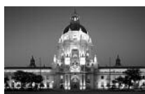
Pasadena City Hall Renovation California, USA
