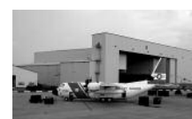
Paint Hangar, Robins Air Force Base Georgia, USA
