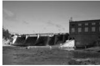
Escanaba No. 3 Hydroelectric Project Michigan, USA
