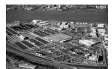
Blue Plains Wastewater Treatment Plant Washington D.C., USA
