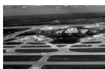
West Airfield Improvements, Orlando International Airport Orlando, USA
