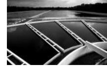
South Austin Regional Wastewater Treatment Plant Texas, USA
