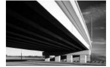
111 St. Bridge / Anthony Henday Drive Edmonton, Canada
