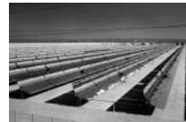
Solar Energy Facility Environmental Consultancy California, USA
