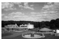
Cheshire Treatment Plant BNR Upgrade Connecticut, USA
