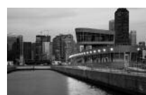
Chicago Lock House Chicago, USA
