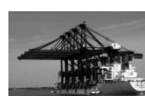
Bayport Container Terminal Texas, USA
