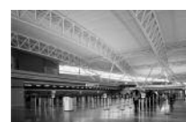
American Airlines Terminal, JFK International Airport New York, USA
