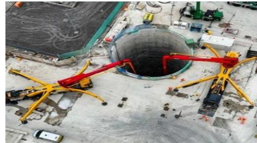
*Delivered innovative solutions to help deliver the world's largest continuous pour of climate-friendly concrete, saving an estimated 82 tons of CO2*
