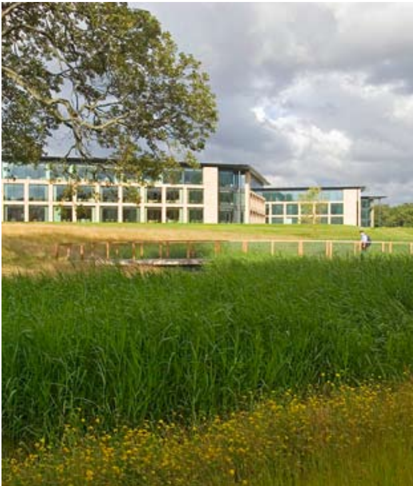
The Royal Bank of Scotland has recently moved into its new 650,000ft 2 world headquarters, just outside Edinburgh. Park land surrounding the offices has been transformed thanks to AECOM's role as landscape masterplanner and designer. Features include a sculptural floodplain to accommodate potential flooding and two large open sustainable urban drainage ponds that have been designed as attractive park land features.
