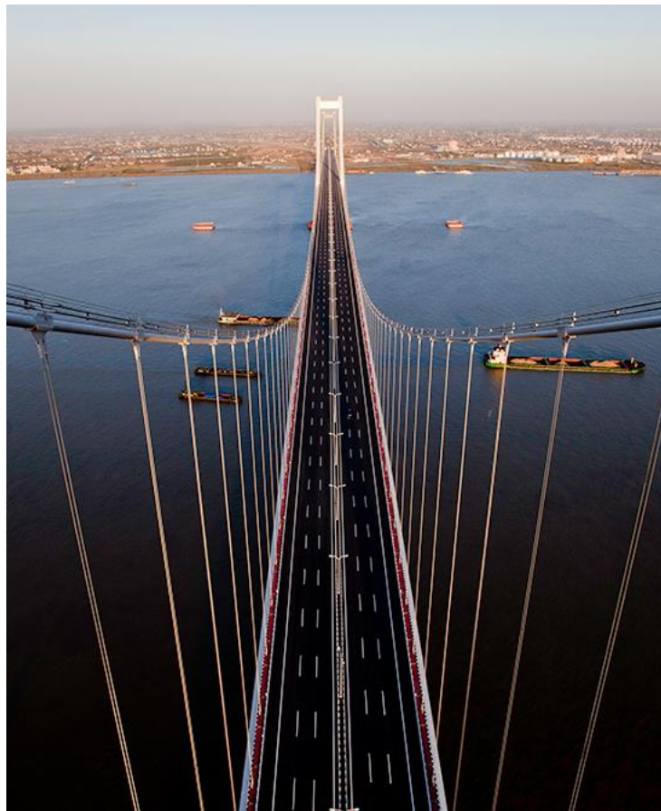
The Taizhou Bridge in Taizhou, Jiangsu, China — the world's first long-span, three-pylon suspension bridge — was presented the Supreme Award for Structural Engineering Excellence from the Institution of Structural Engineers.
