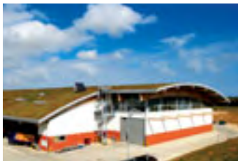
Adnams Distribution Centre Suffolk, U.K.
