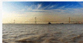
Taizhou Bridge construction, Jiangsu Province, China
