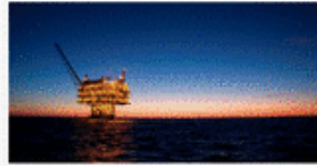
Environmental Licensing Services for Offshore Operations, Rio de Janeiro, Brazil
