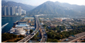
Relocation of Sha Tin Sewage Treatment Works to Caverns in Hong Kong
