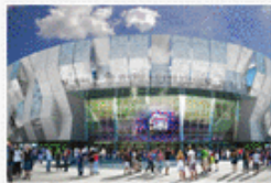
Sacramento Kings Arena - AECOM
