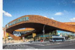
Barclays Center, Brooklyn - AECOM
