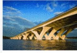
Woodrow Wilson Bridge Project - URS
